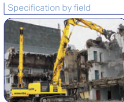
High reach demolition
